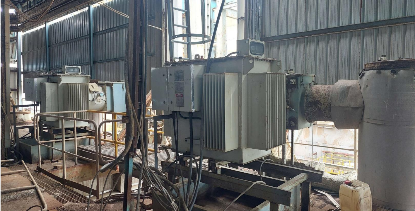
Old 1-Phase Transformers installed in all remaining Fields to be replaced in phase manner
