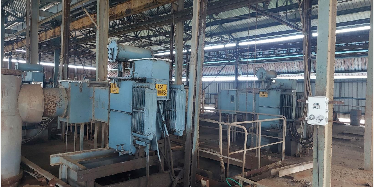
Old 1-Phase Transformers installed in all remaining Fields to be replaced in phase manner
